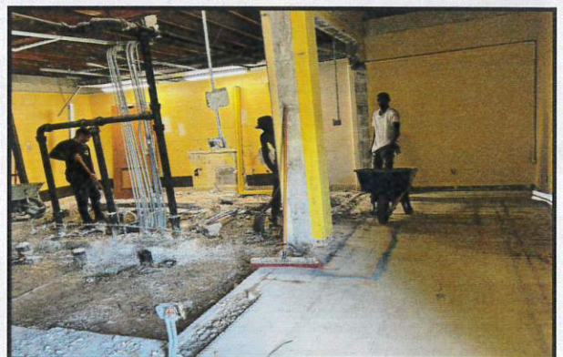
Work in Progress in the Ladies & Men's Restrooms
